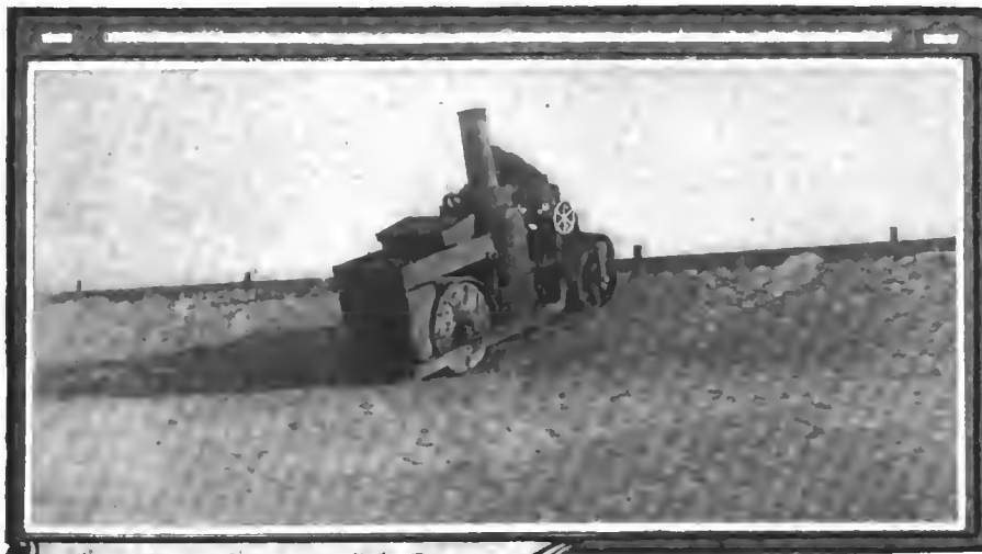
15-Ton Roller up 36 Degree Embankment
